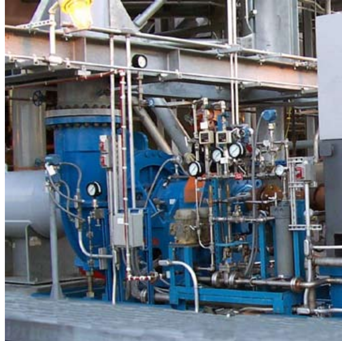
Hazleton CTC 20-30 with 20" suction and discharge
